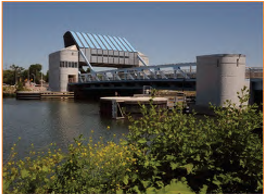
FORT STREET BRIDGE, DETROIT, MICHIGAN
